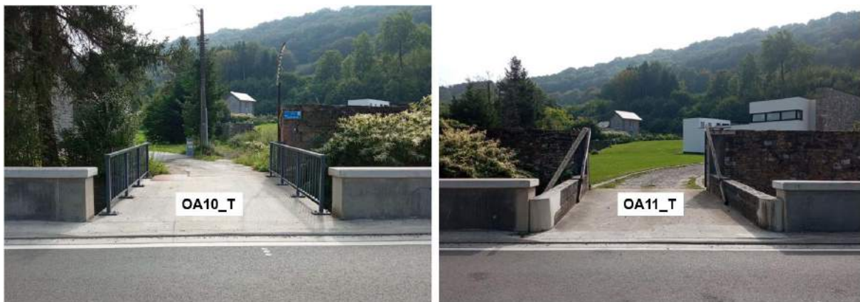
Figure 5-26 : Photos showing the location of structures OA10_T and OA11_T
