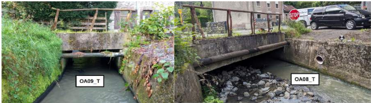
Figure 5-23 : Photos showing the upstream end of structures OA08_T and OA09_T
