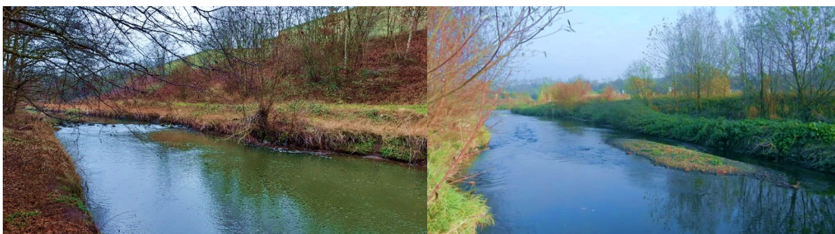
Figure 3.1 Left depicts the current situation with a wide and uniform summer bed and a stone-filled bottom trap, while on the right, the intended situation shows micro-meandering/narrowing of the summer bed achieved through a gravel bank.
