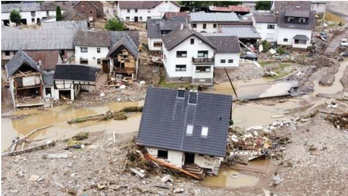
Figure 1: Flood damages in Schuld, Germany (Source: Reuters).
