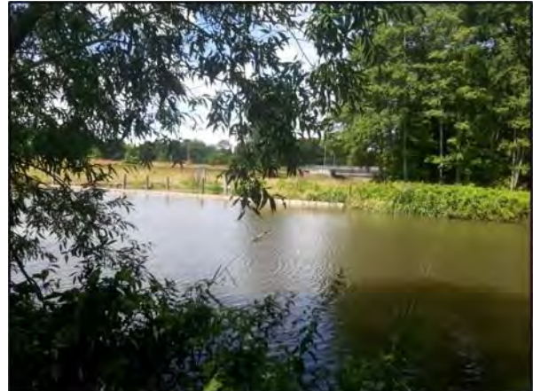
Plate 2. Upstream inlet to the bypass channel which has poles and a boom to prevent floating debris from entering.
