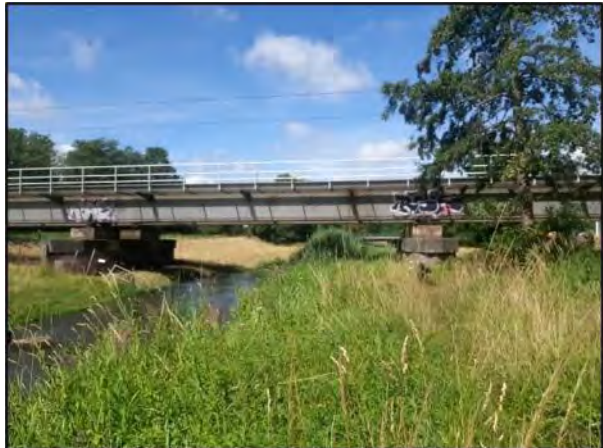
Plate 4. View downstream along the Groene Overlaat channel to the railway bridge.
