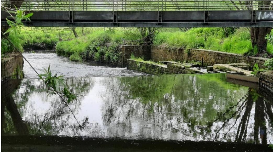
Figure 1.3 Photo of the Geul at station Sippenaeken at low discharge on 15 May 2023, with a downstream view of the weir, a fish ladder, a gate to a side channel and a pedestrian bridge.
